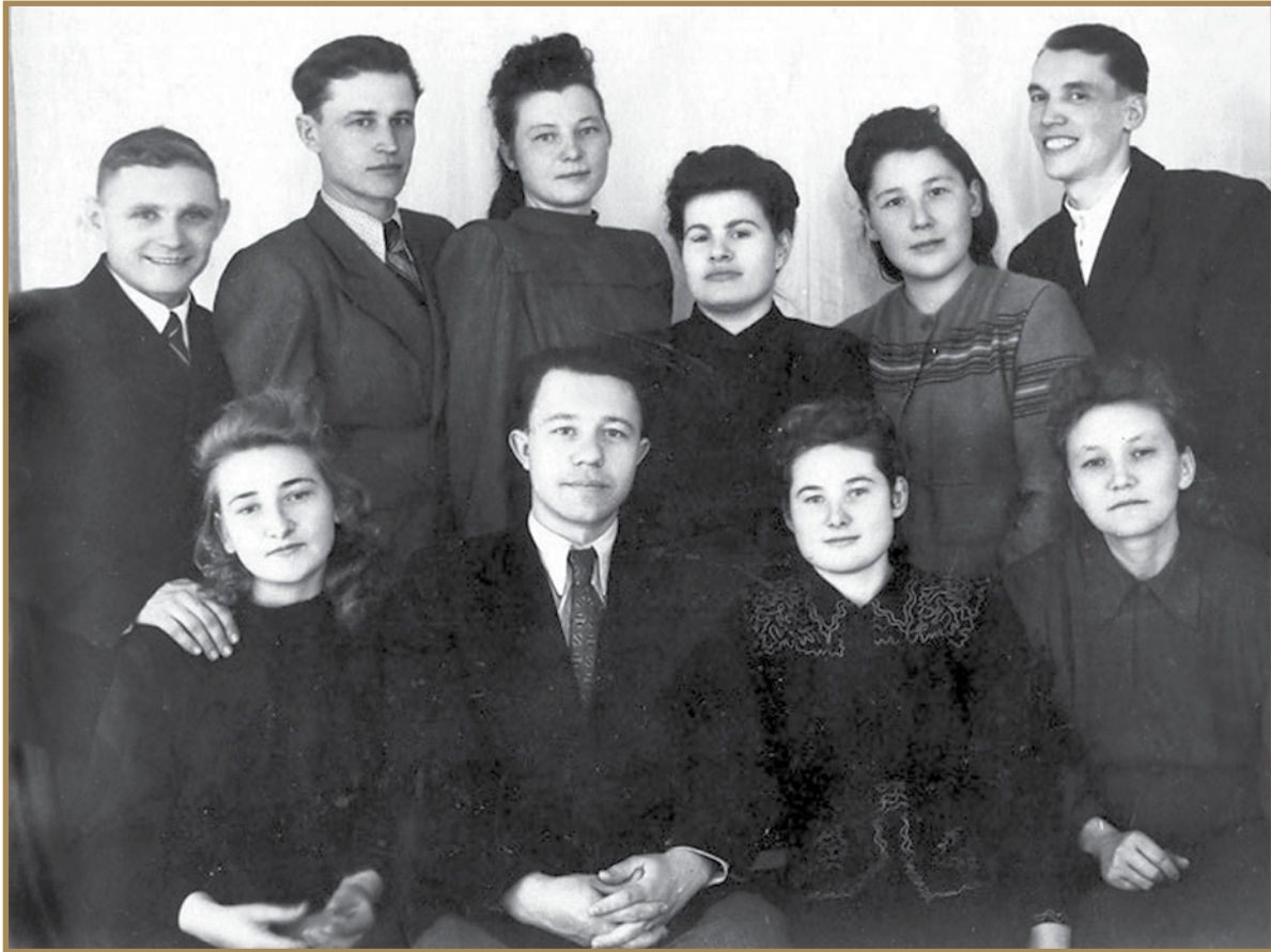
ЖЭО ұжымы Коллектив ТЭЦ Central Heating and Power Plant employees
